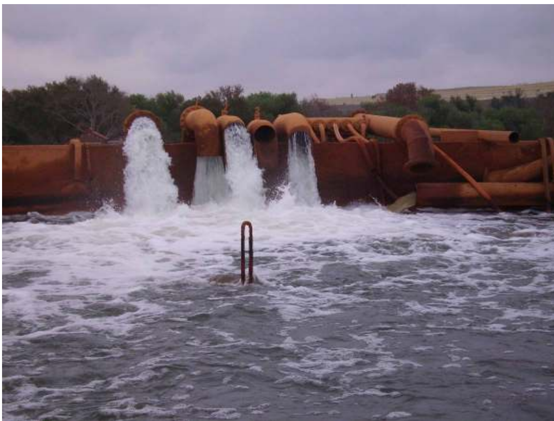
Figure 4.4. Water pumped from the Eastern Basin to the treatment plant at Grootvlei Mine
